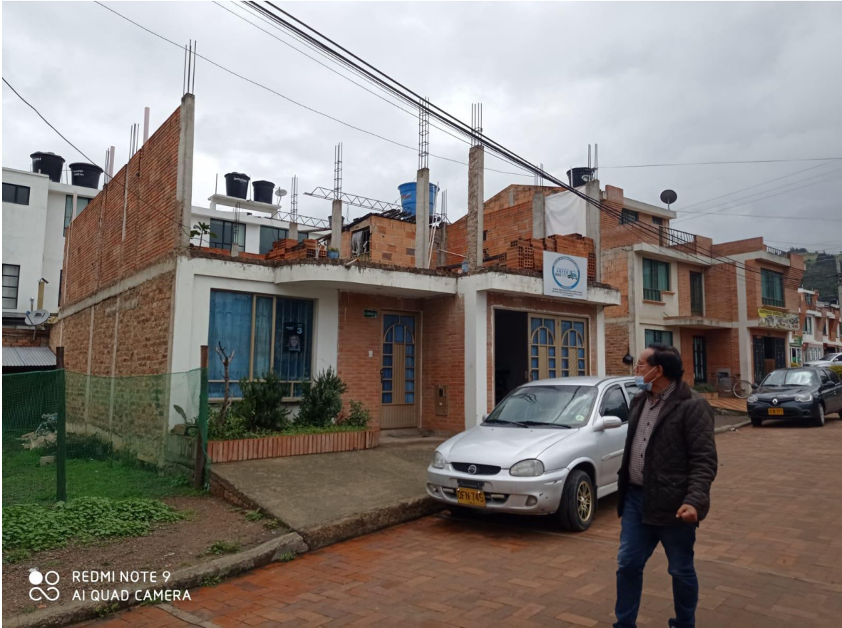
Vista fachada principal
