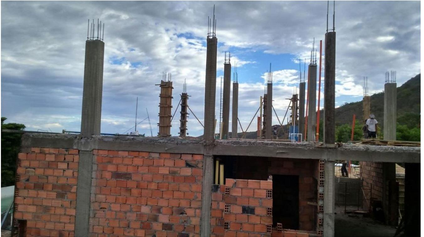
COLUMNAS Y VIGAS CON REFUERZO
