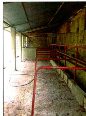
INTERIOR ESTABLO –CA19.
